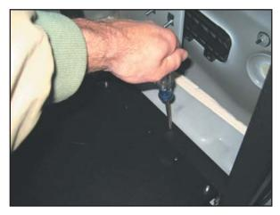
Attach bottom frame with three (3) - # 10 x 3/4" sheet metal screws.
